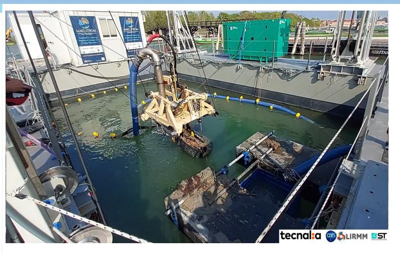
Realtime RTK-GPS positionning to move the robot and gripper above the target and dive
